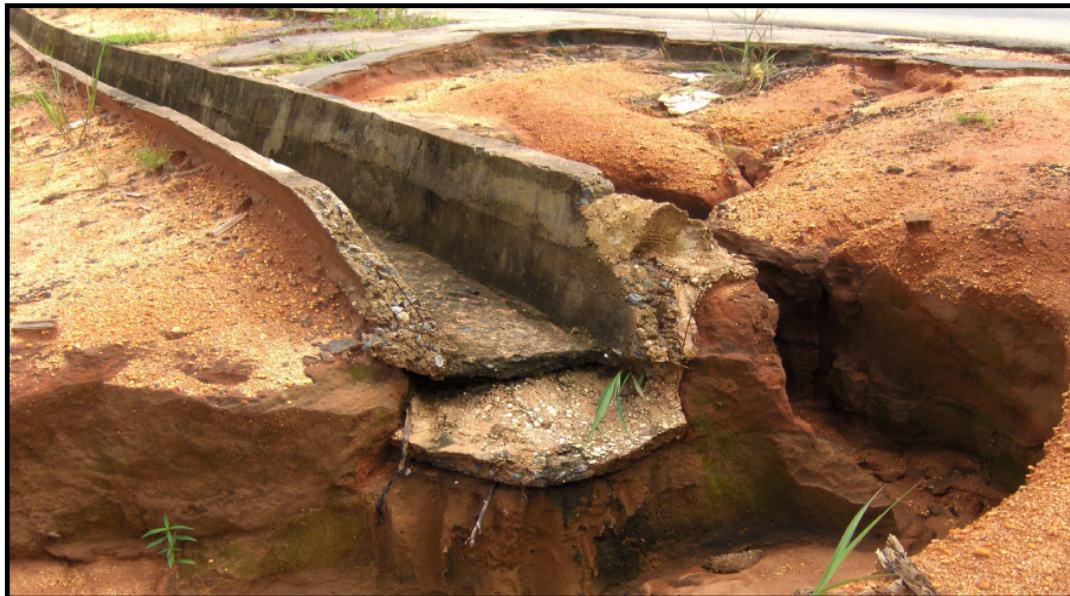
Figure 7: Improper termination of drainage channel forming gully erosion triggers.
