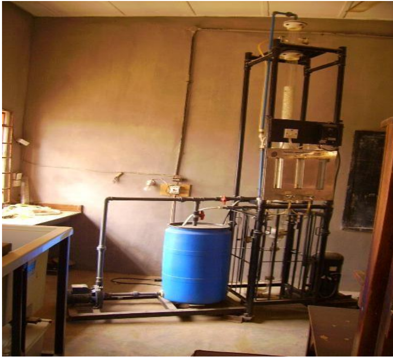
FigureG-1a: The photograph of the prototype pilot plant packed absorption tower before renovation and upgrade.
